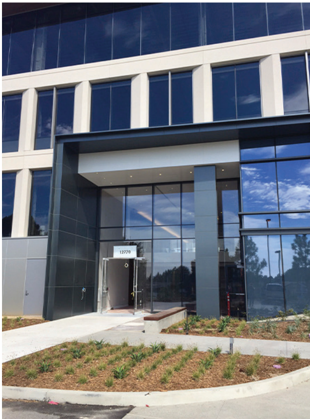
Figure 4.4a Precedent photo of building entry
